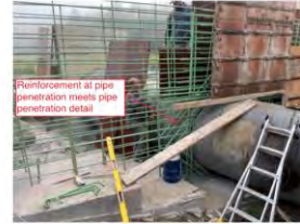
Photo 1: Cutoff wall epoxy coated reinforcing steel placement completed. Formwork in progress.
