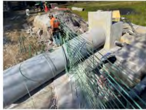
Photo 3: Epoxy coated reinforcing steel from above.
