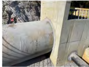
Photo 4: 48-inch RCP and steel low-level outlet pipe grouted into outlet structure
